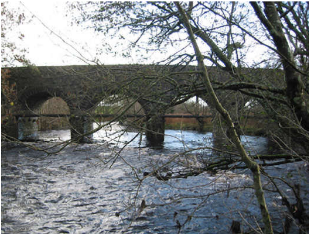
Plate 13.88: NIAH Reg. 31302109 Tonrehowan Bridge (photo courtesy of www.buildingsofireland.ie ).
